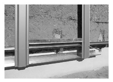
When using the DEKMETAL load-bearing construction, the same principles apply to the spacing of vertical profiles and anchoring elements – see the table of the Maximum axial distances of anchoring elements in chapters 7.1.3.1 Application of the CETRIS<sup>®</sup> VARIO boards and 7.1.3.2 Application of CETRIS<sup>®</sup> PLANK boards.
